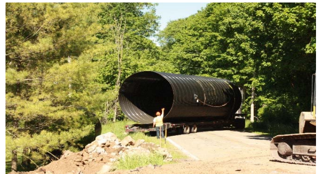
Musgrove Hwy culvert
